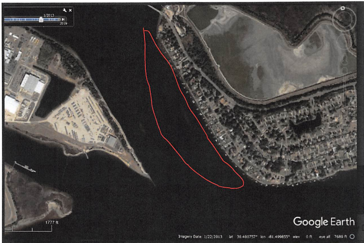
Figure 3. Shoaling in the area of the confluence of Clapboard Creek and the St. Johns River. The shoaling is approximated in red. Additional shoaling is occurring to the Northwest on the opposite side of the mouth of Clapboard Creek.
